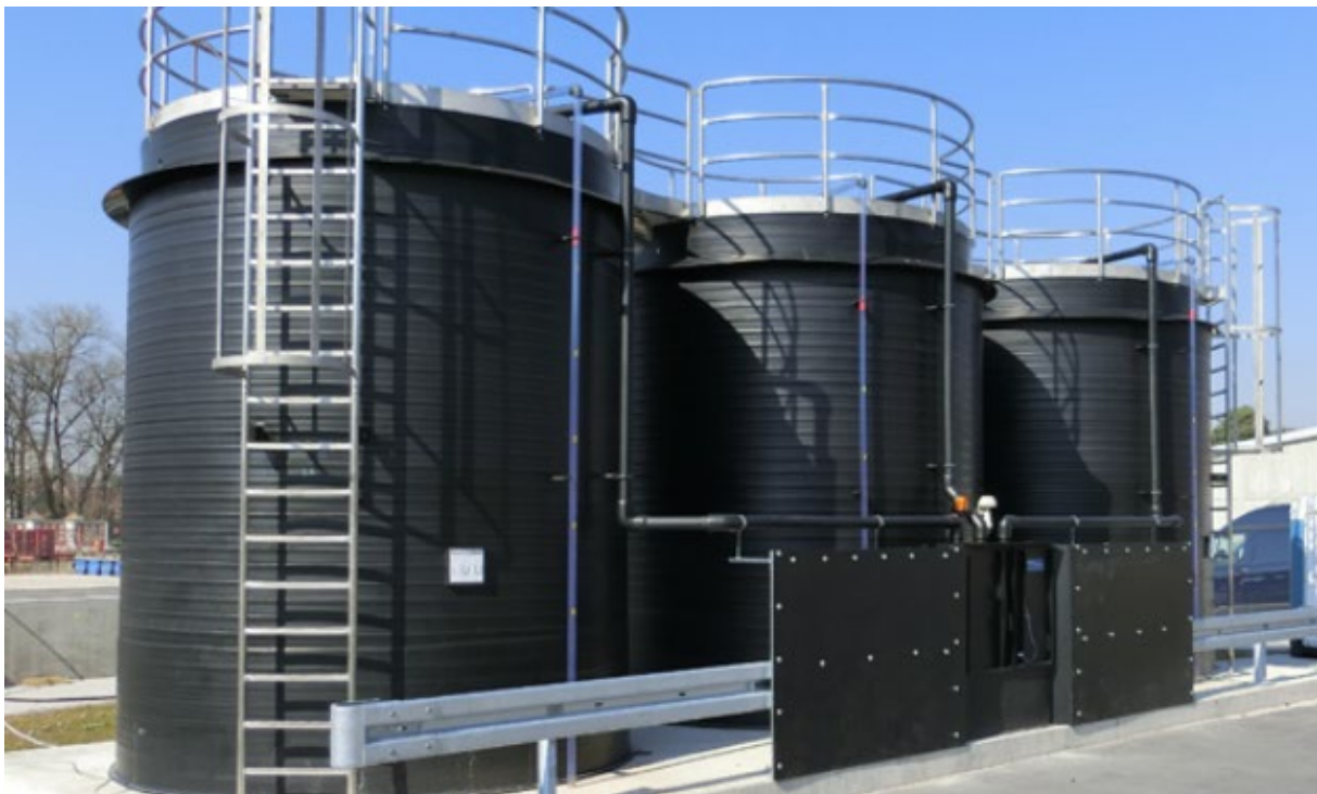
Figure 2-39: Double-walled HDPE tanks 40
