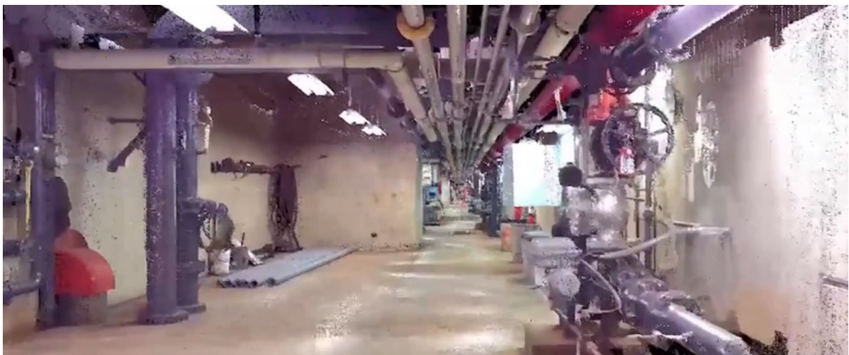
Figure 1-28: Autodesk Recap® 3D Laser scanning view of a pipe route
