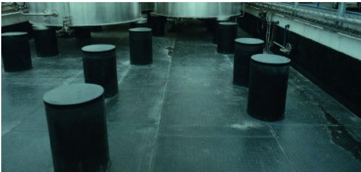
Figure 2-38: Collection tray coated with HDPE 39
