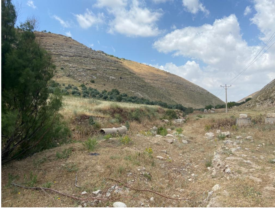
Figure 3: Segment of the pipeline route
