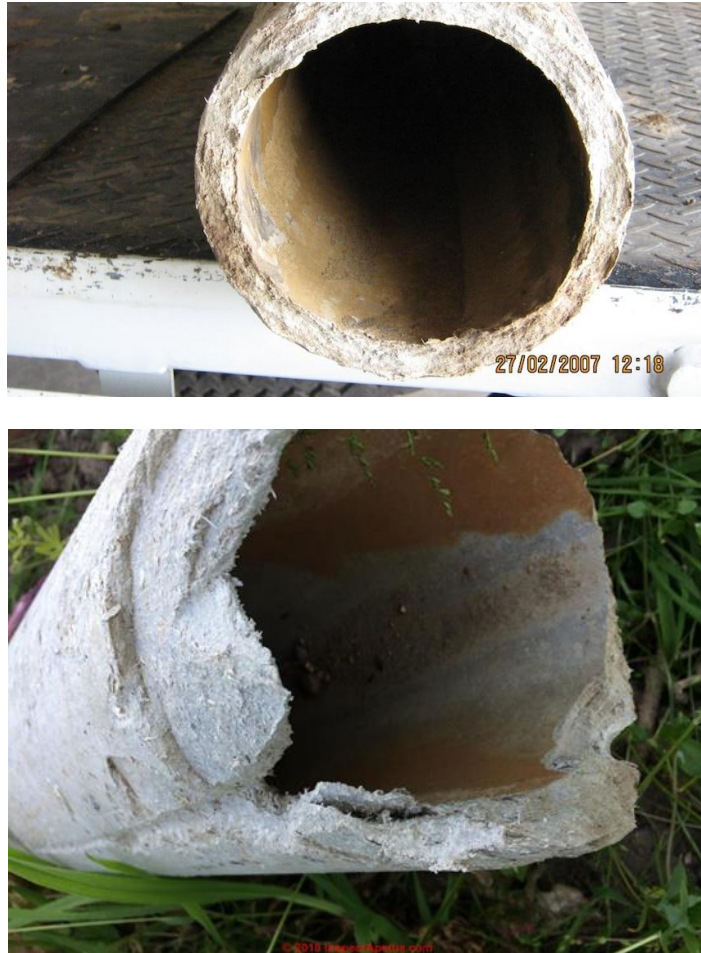
Figure 6:Old Water Pipes
