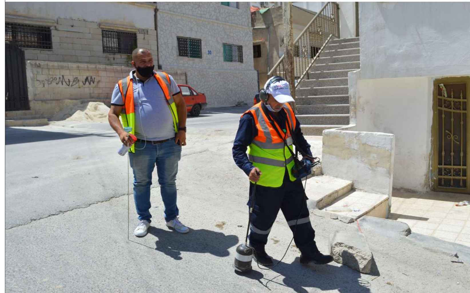
Leak detection in Miyahuna
