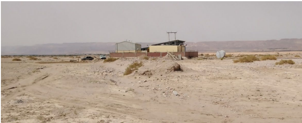
Figure 1-15: Rahma BWRO plant
