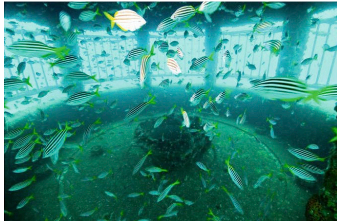
Velocity cap intake during operation
