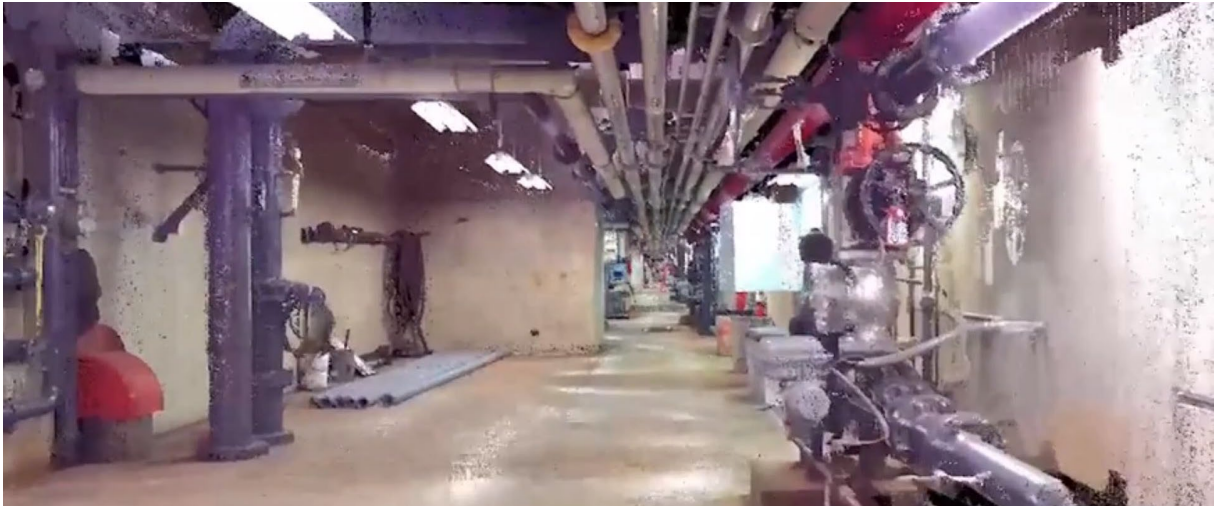
Figure 1-19: Autodesk Recap® 3D laser scanning view of a pipe route
