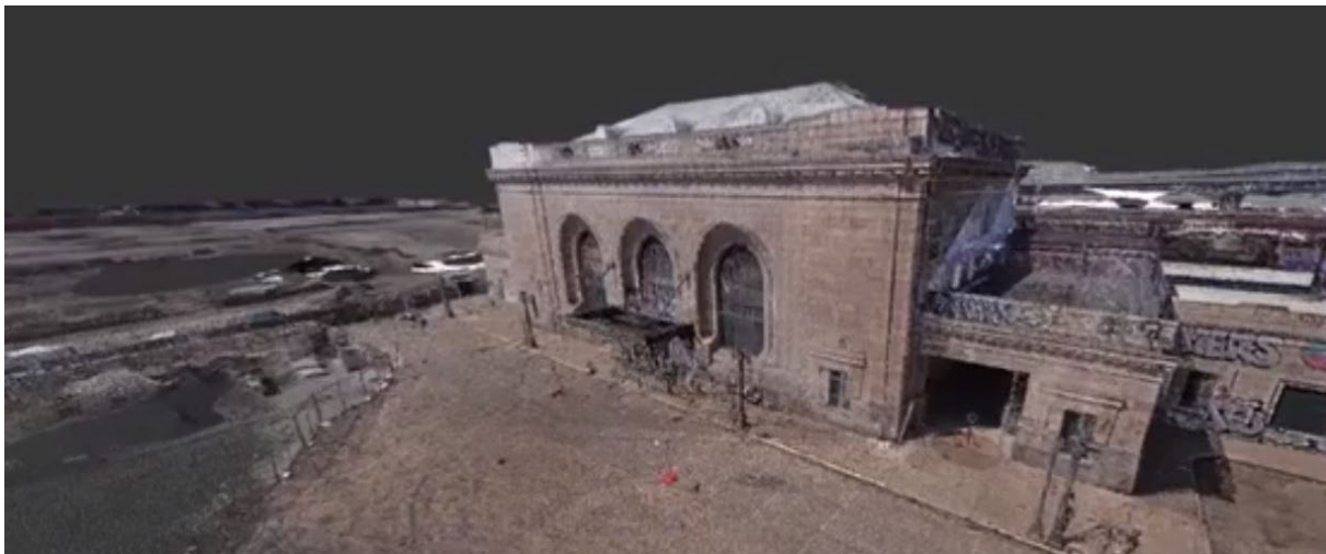
Figure 1-18: Autodesk Recap® 3D laser scanning view of a building
