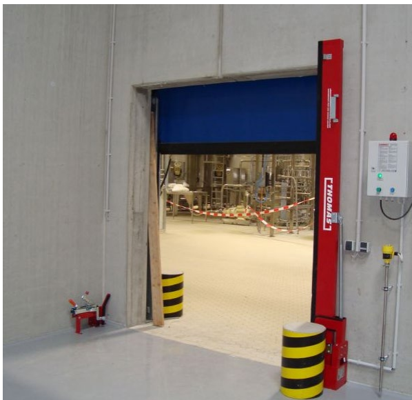
Figure 2-62: Extinguishing water retention barriers 39
